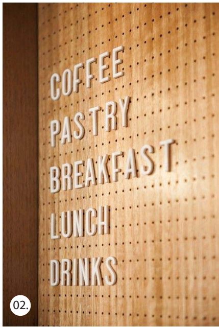
01. PLY CLAD SEATING & PENDANTS LIGHTING OVER 02. PIN BOARD MENU WITH WHITE ACRYLIC PUSH FIT LETTERING 03. BUILT IN BENCH SEATING & UPHOLSTERED CUSHIONS 04. TIERED DONUT GLASS DISPLAY 05. PLY CLAD COUNTERFRONT 06. WHITE NEON BRANDING 07. UNIFORMS 08. RECONSTITUTED STONE COUNTER TOPS 09. COLOURFUL FURNITURE 10. GELATO DISPLAY 11. ROUNDED TIMBER TABLE TOPS
